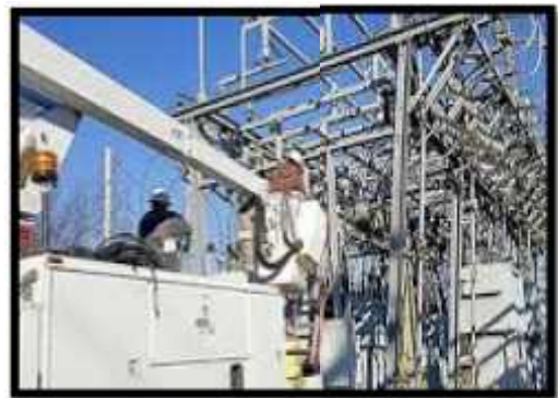
City crews working on substation two, Saturday morning.
