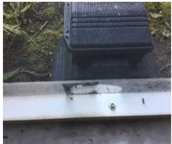
Rats have chewed through the screen of a lanai at a home in the Village of Bonnybrook.
